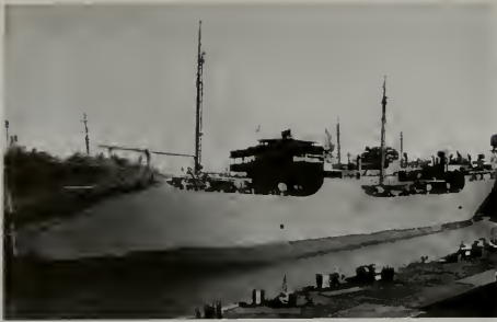
The Mobilube, her torpedo damage repaired, is shown above at dock prior to being drydocked for installation of tail shaft and wheel.
